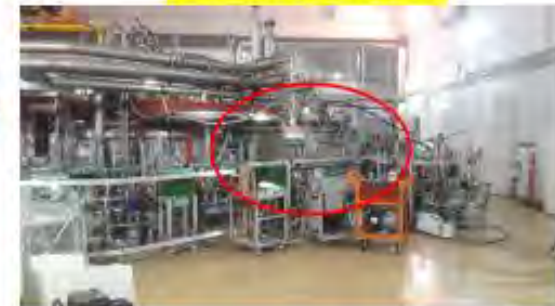
RIB LINAC AT VECC
