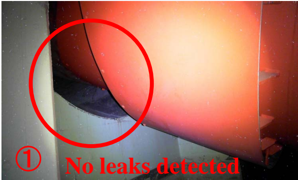
Vent pipe sleeve end
