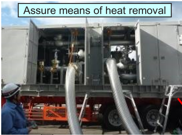
Turbine Water Lubricant pump
