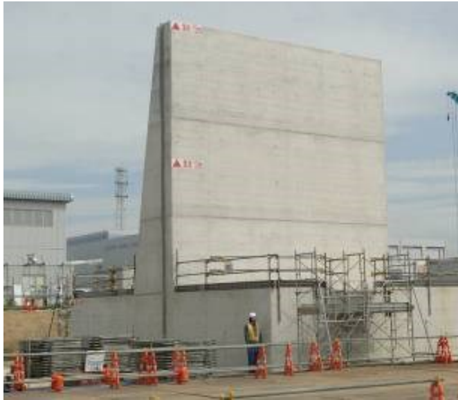
Embankment : Preventing inundation of site
