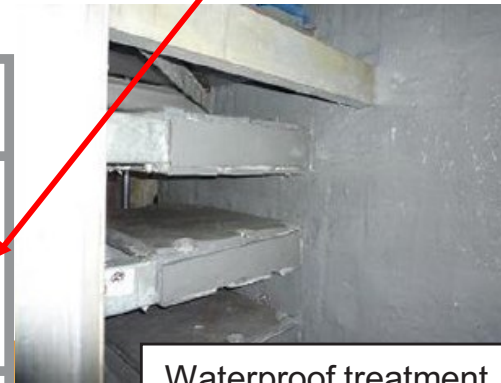
Waterproof treatment at Cable trays
