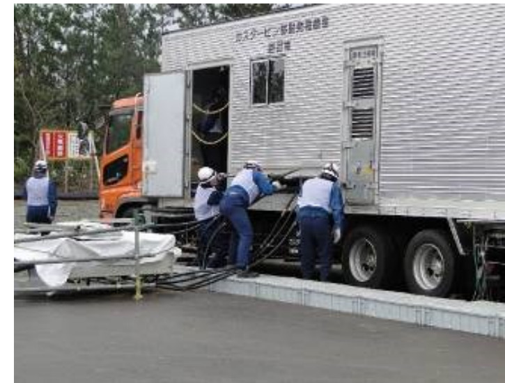
GTG connection drill
