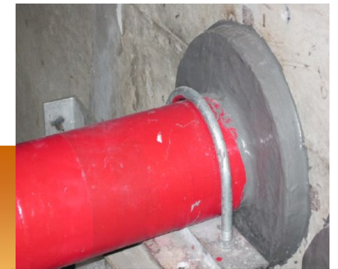
Waterproof treatment at Pipes
