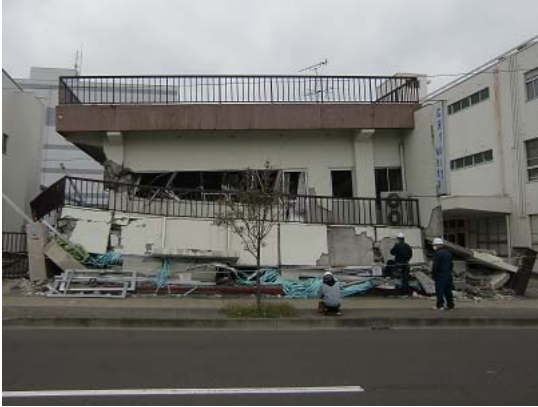
Collapse of First Story in Two-Story RC
