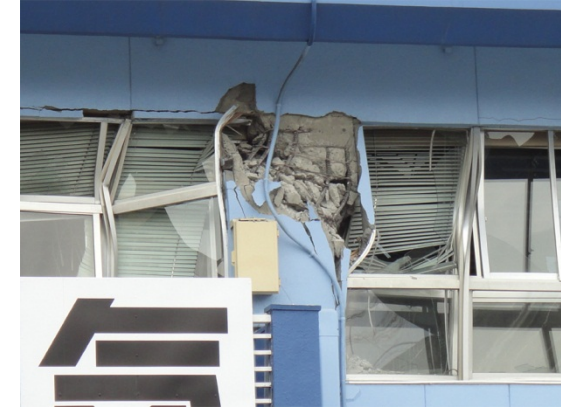
Shear Failure of RC Columns
