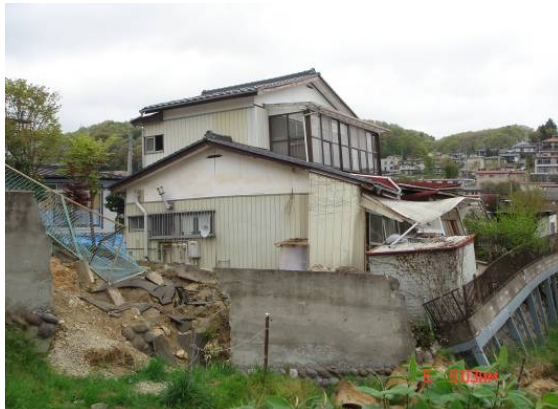
Failure of House by Landslide
