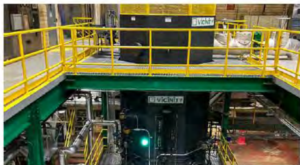
42MW Electric boiler
