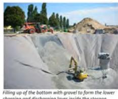
Filling up of the bottom with gravel to form the lower charging and discharging layer inside the storage.
