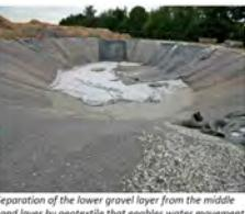
Separation of the lower gravel layer from the middle sand layer by geotextile that enables water movement and protect the gravel from sand intrusion.
