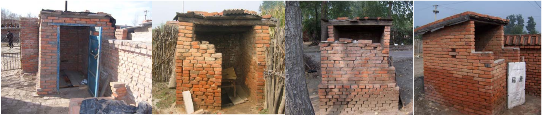
Brick and concrete
