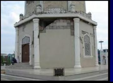
Severe cracking and spalling of concrete
