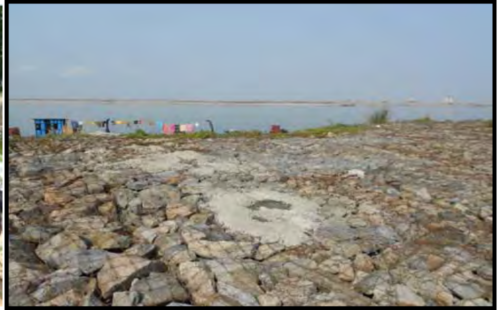
Anti- erosion work with wire-mesh of Stone
