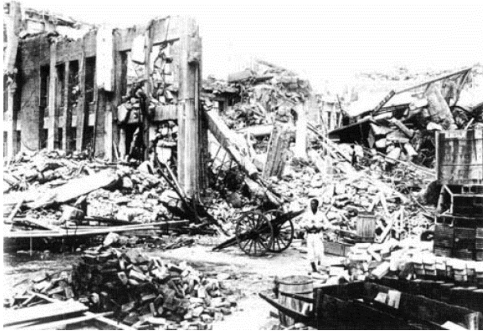
Naigai Bldg. (collapsed during construction)
