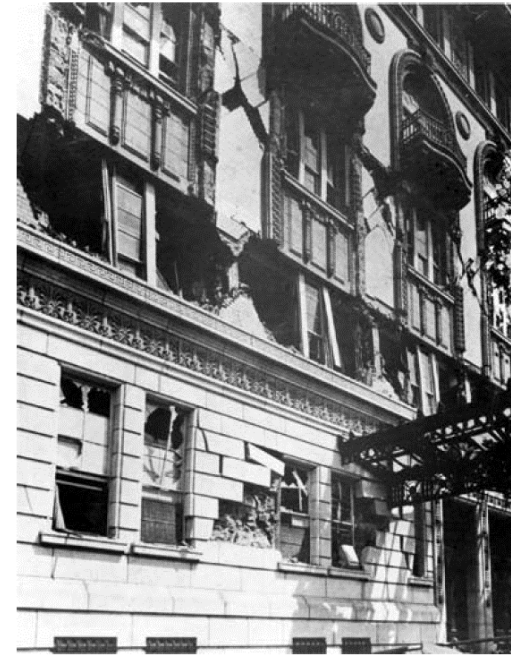
Tokyo Kaikan Bldg. (built in 1922)
