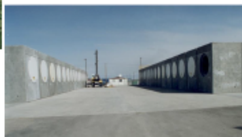
2000 – 2001 Removed from pool, dewatered, dried, and placed in dry storage
