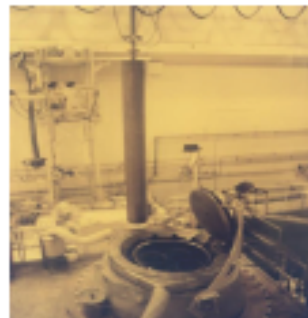
Loading a Canister into the Vacuum Dryer
