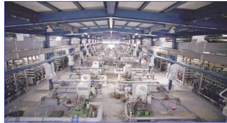
RO building area, UAE
