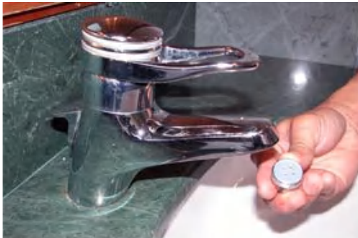
Installation of Thimble
