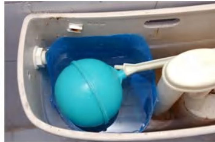
Installation of cistern water saving bag
