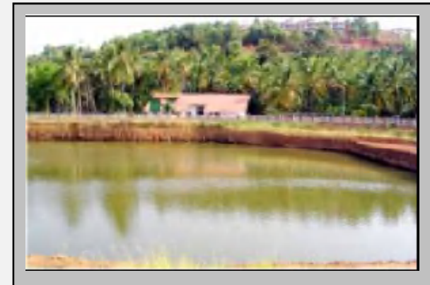
The large pond that stores rainwater for the campus.(30 million litres capacity)
