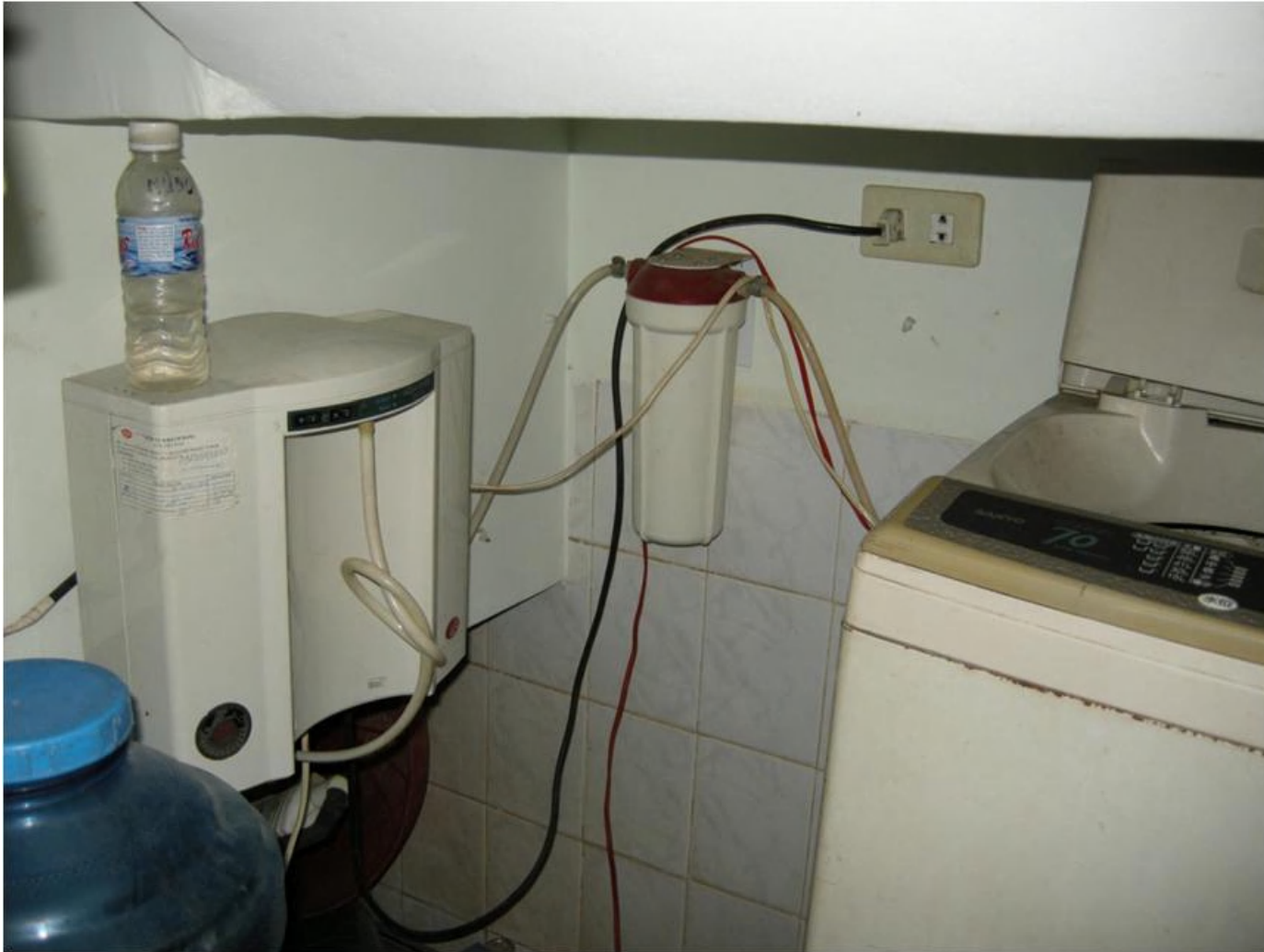
Groundwater purification system in household (Ho Chi Minh City)
