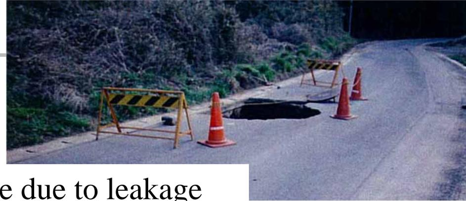
Subsidence due to leakage
